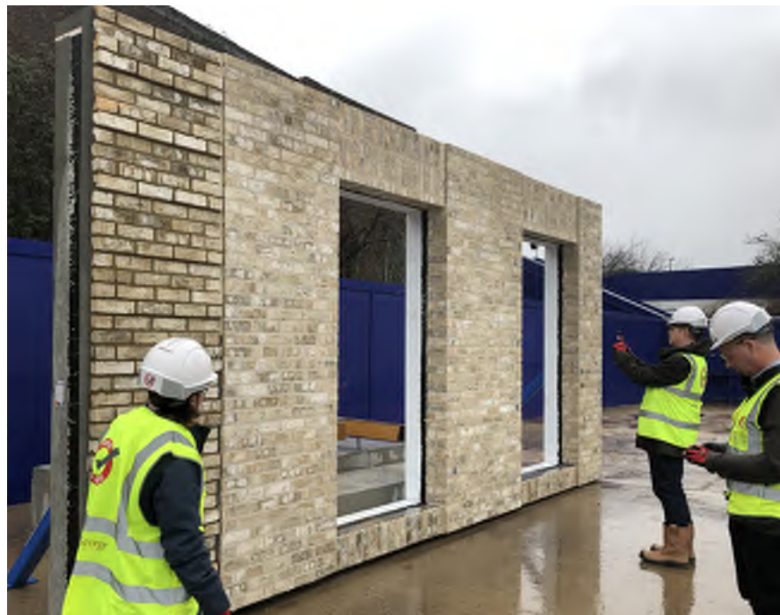
PHASE 1 - BRICK CLADDING SAMPLE PANEL
